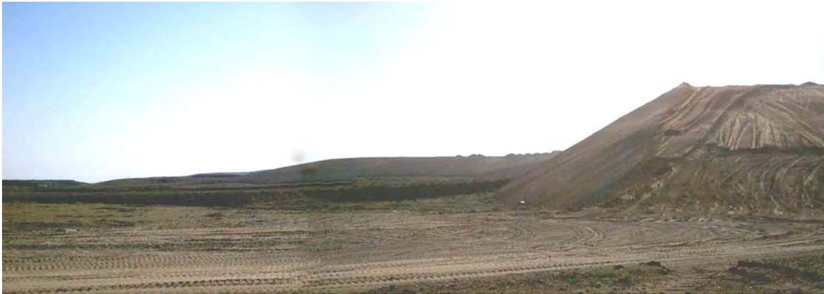
*Fig. 2. Rehabilitated dump on the East Mine which stockpiled 2,000 tons of radioactive metal structures and now makes them inaccessible for extraction and reuse. (Source KAEC Kazakhstan)*
